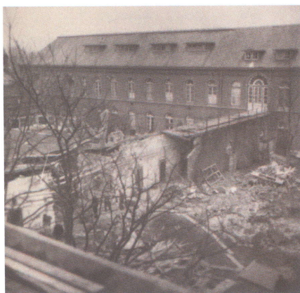
Schade door bom in 1945.
